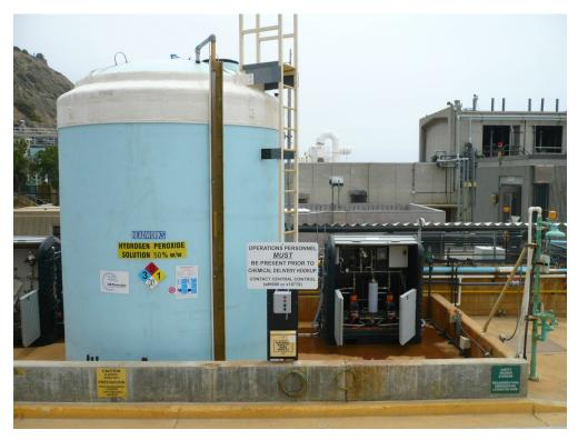
Figure 6: Headworks Hydrogen Peroxide Feed System
