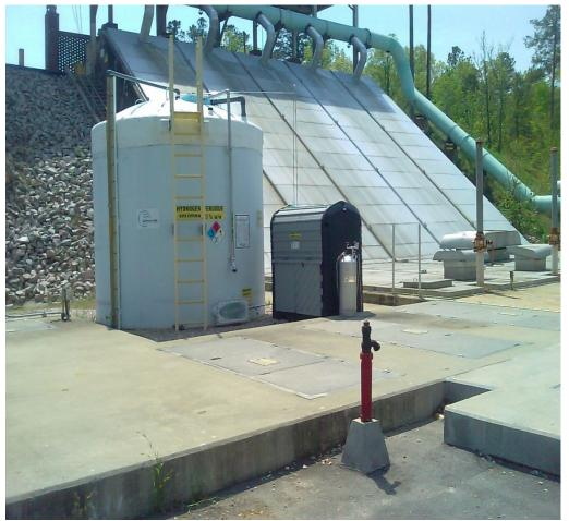
Figure 4. Hydrogen Peroxide System Installation at Walnut Creek Lift Station
