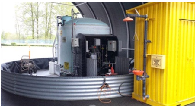
USP's Peracetic Acid Bulk Equipment and Safety Station
