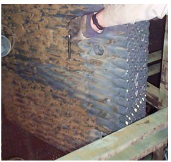
Figure 36. Fouling is light for the first 6-12 inches down into the fill pack due to higher water velocities at the top.
