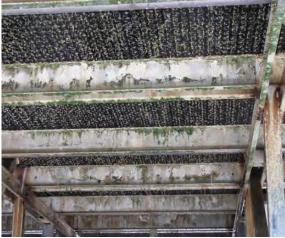
Figure 23. Tower fill pack from bottom prior to peroxide cleaning.
