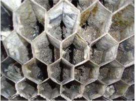
Figure 9. Scaled wet-dry interface area of integral louver fill
