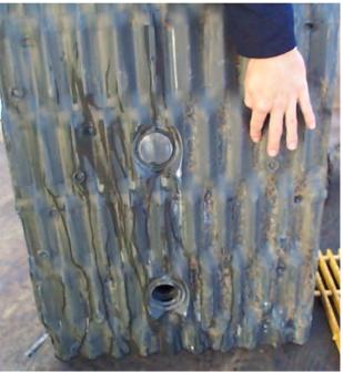
Figure 39. Tower fill close-up after cleaning showing essentially complete deposit removal.
