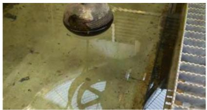
Figure 34. Tower sump after flushing
