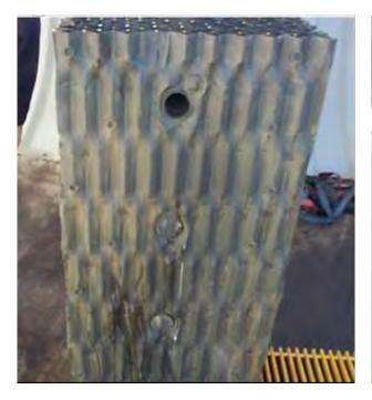
Figure 38. Tower fill section after peroxide cleaning.
