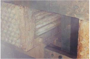
Figure 12. "Coil shed" tube bundle showing tube OD's encased in a thick layer of white calcium carbonate at the start of the cleaning
