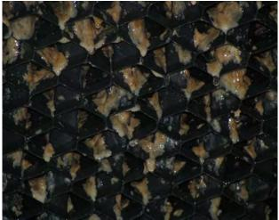
Figure 25. Close-up of underside of fill pack prior to peroxide cleaning showing gooey slime buildup.
