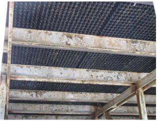
Figure 24. Tower pack after peroxide cleaning.
