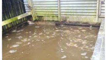
Figure 33. Tower sump of same cross-flow tower during peroxide cleaning. Peroxide is very effective at dislodging biofilm-silt deposit matrices.
