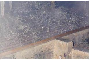
Figure 13. Tube bundle totally white with calcium carbonate under a spray nozzle near the start of the cleaning procedure
