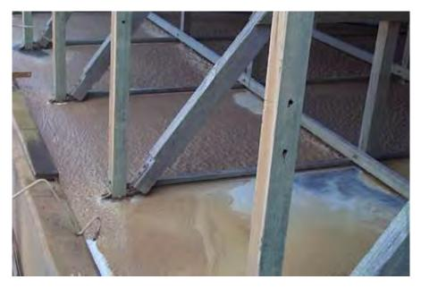
Figure 40. Tower sump with cell off line after cleaning showing some of the dislodged dirt floated to the surface by peroxide micro-bubbles.
