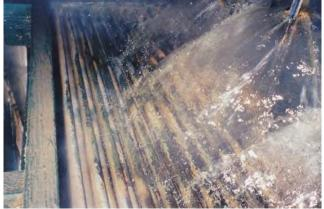
Figure 14. Tube bundle showing some bare tube metal part way through the cleaning procedure.
