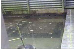
Figure 32. Tower sump of heavily fouled industrial cross flow film fill tower prior to peroxide cleaning
