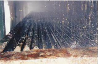
Figure 15. Tube bundle at the completion of the cleaning process showing mostly bare tubes.
