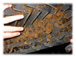
Figure 6. Fouled cross-fluted fill that is no longer highly efficient
