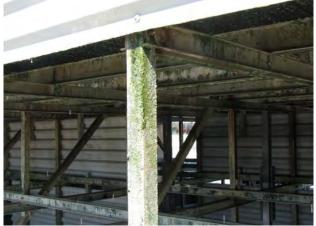
Figure 27. Structural supports prior to peroxide cleaning showing some green algae buildup.
