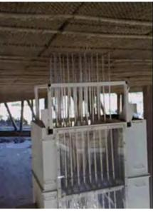
Figure 16. Mechanical cleaning apparatus for calcite scale on a natural draft tower.
