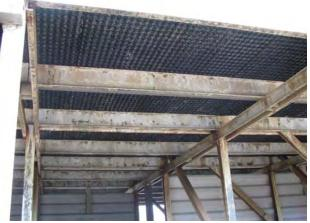
Figure 28. Structural supports after peroxide cleaning showing algae substantially bleached and removed.
