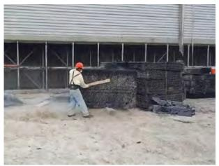
Figure 17. Forehand mechanical cleaning technique for silica scales.
